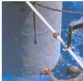
Spreading of SUBCOM T.260 on steel piles
